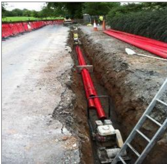
Figure 3 - 110kV Underground Duct Installation
