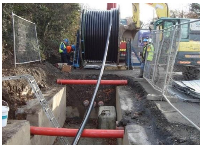
Figure 12 - Typical Cable Pulling Drum Set Up
