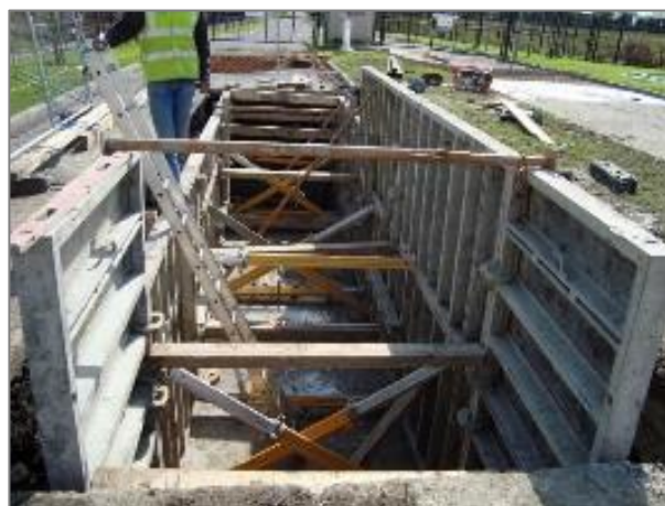
Figure 9 - Typical joint bay under construction (in-situ)
