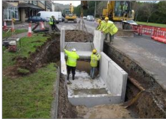
Figure 11 - Typical joint bay under construction (pre-cast)
